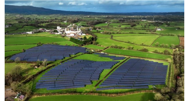
Astatine 5MW Dale Farm Installation
